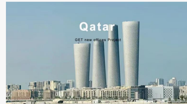
Qatar GET Office Building Project
