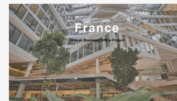
France Orange Business Office Building Project
