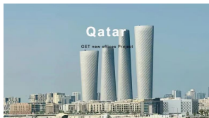
Qatar GET Office Building Project
