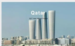
Qatar GET Office Building Project
