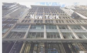
US SIONI GROUP Office Building Project
