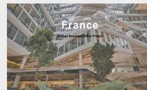
France Orange Business Office Building Project
